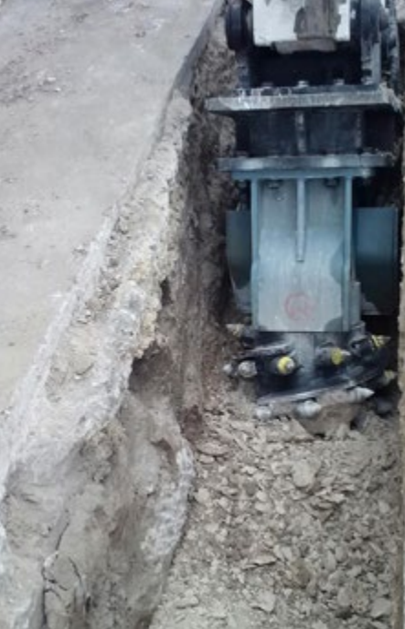
TC20 Digging a Utility Trench
